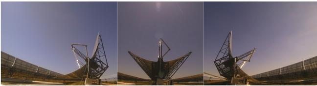
Figure 1: Example of solar tracking in a real PTC.
